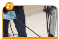
Wind cable back into handle, wiping clean with a damp cloth as you do.
